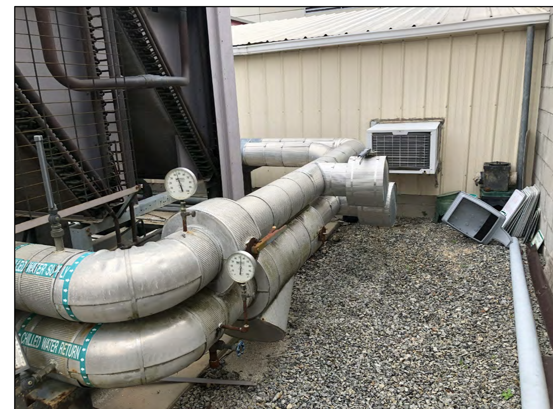
② PHOTO OF EXISTING CHILLED WATER PIPING NTS
