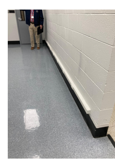
2. EXISTING ELECTRICAL RACEWAY IN HALLWAY 304
